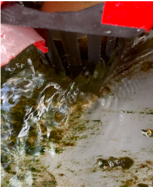
Figure 14. The large biomatter buildup that suffocated Plant 7 in the Pipe System. Note how the biomatter is clogging the basket.
